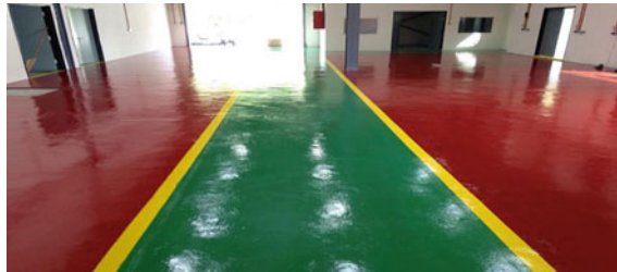
Fig. 4 Epoxide resin paint used as finishing for the laboratory’s floorings
