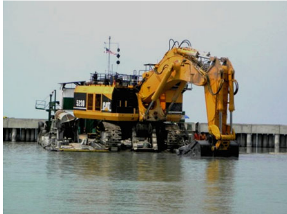
Fig. 2 Backhoe dredger at work in the Marina Melaka, Melaka
