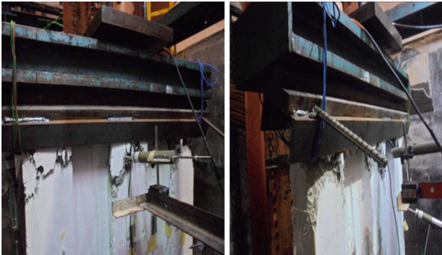
Fig. 13 Crushing failure occurred at the top of three-ribbed WSF wall
