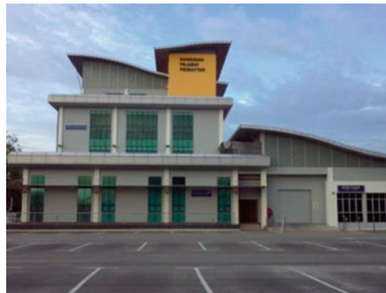
Fig. 4 Registrar office building (side view)
