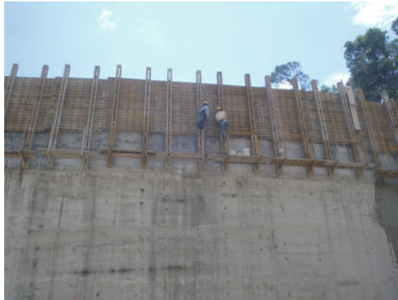
Fig. 3 Carpenter fixing the formworks at upstream of the dam
