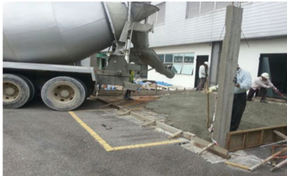
Fig. 6 Pouring of G25 concrete to gas compressor house ground floor slab
