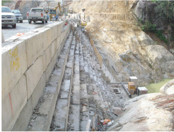
Fig. 4 Concrete block are arrange to form a 600 m downstream step
