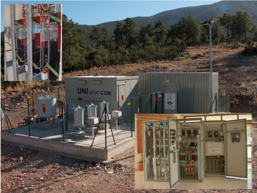
Fig. 12.2 STATCOM prototype in Turkish transmission system
