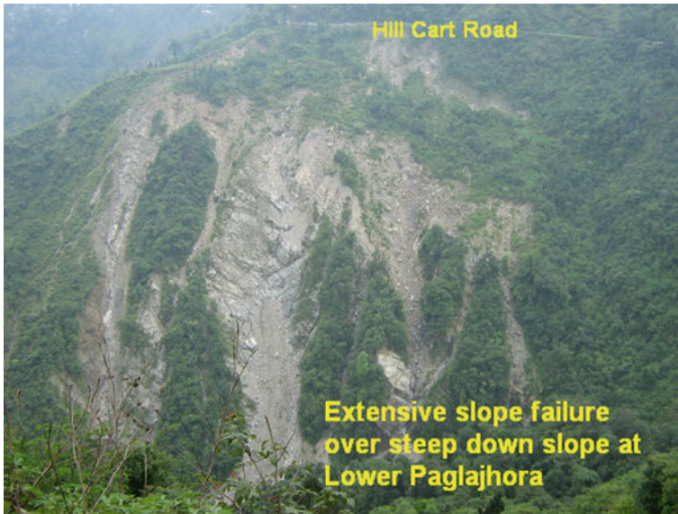
Fig. 8.14 Massive landslide at Paglajhora
