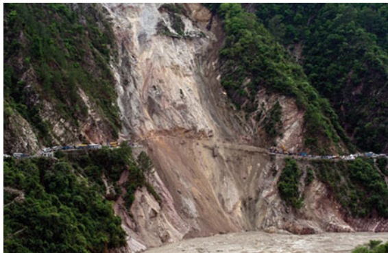
Fig. 1.9 Elimination of road by landslide, Kedarnath (Source www.srinistuff.com )
