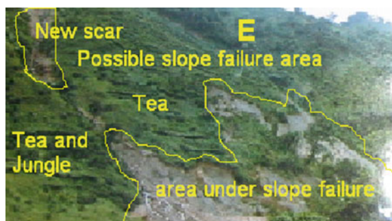
Fig. 1.18 Massive damage of tea estate, Shiviter
