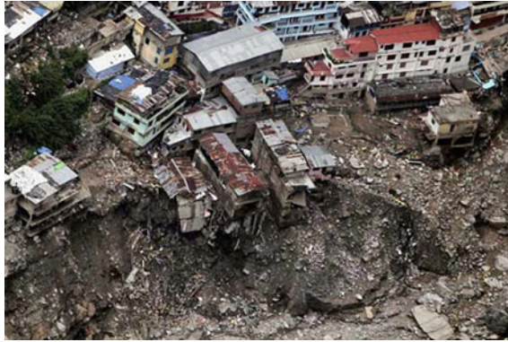
Fig. 1.8 Slope failure and destruction of settlement at Kedarnath ( www.dailymail.co.uk )
