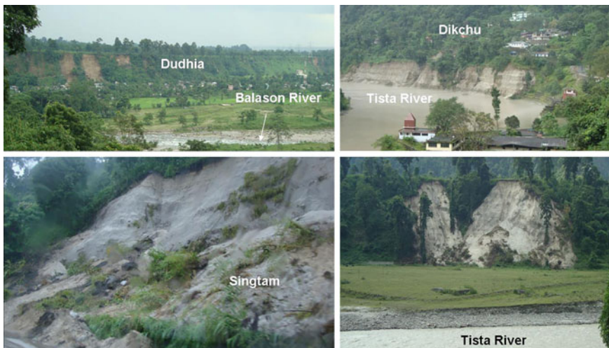
Fig. 1.5 Some fresh landslides after Sikkim Earthquake, 2011 (Source GSI, Engineering Division, Gangtok)
