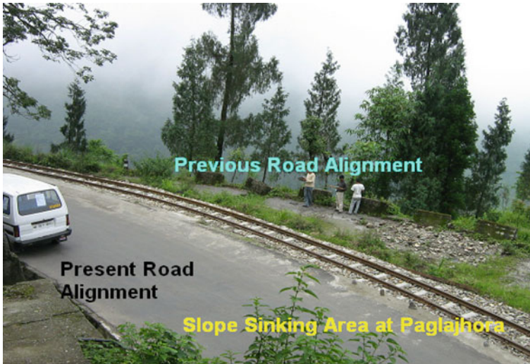
Fig. 8.20 Reconstruction of the Hill Cart Road near Paglajhora
