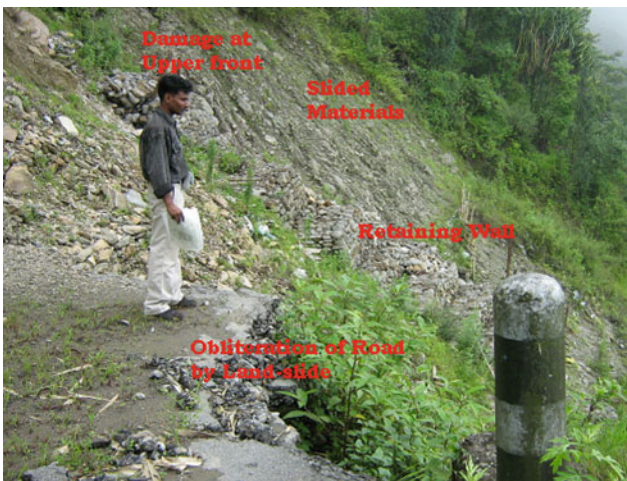
Fig. 8.6 Retaining wall at lower Paglajhora
