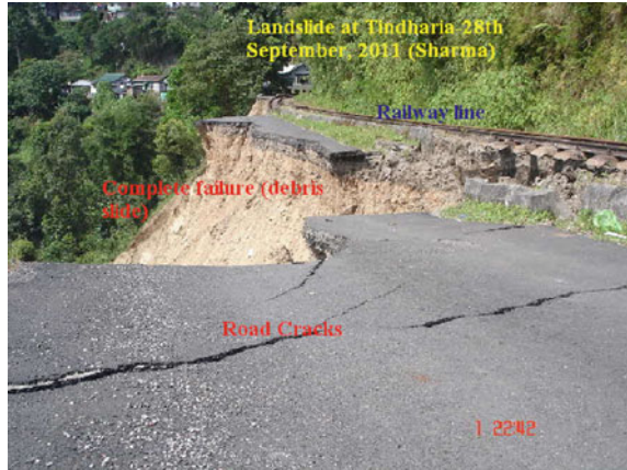
Fig. 1.15 Road damage at Tindharia
