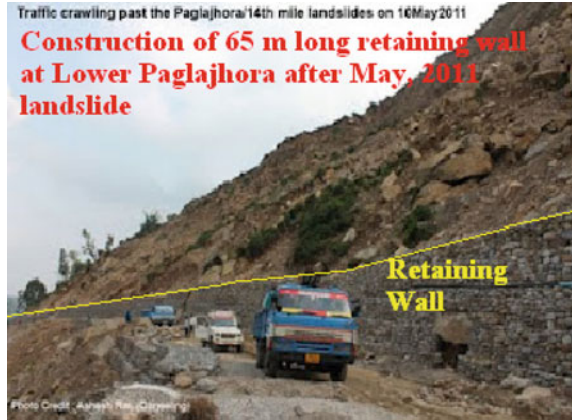
Fig. 8.8 Retaining wall at lower Paglajhora
