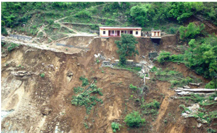
Fig. 1.11 Down ward movement of fragile slope materials (Source www.dailymail.co.uk )
