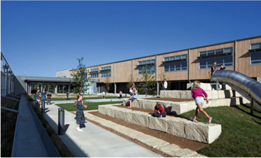
Fig. 2 The Kiowa County Schools designed by BNIM Architects (Photograph by Assassi)
