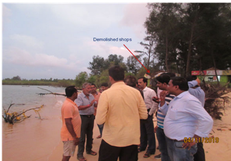
Photo 1 Image showing the demolished shop
