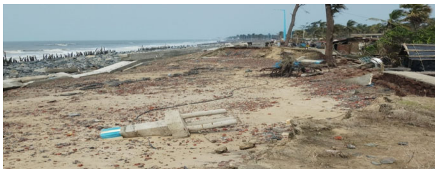
Fig. 4 Guard wall damaged and black top road behind damaged, washed out at Jaldah as observed on 28.5.2021
