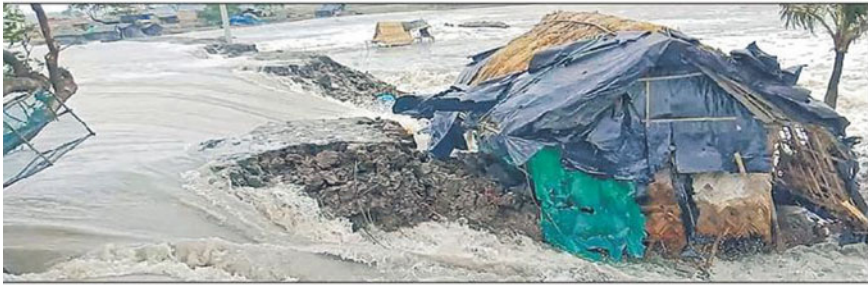
Fig. 13 Flood in Uttarmamudpur of Hingalganj of South 24 Parganas district due to embankment breach of Icchamati river as observed on 26.5.2021
