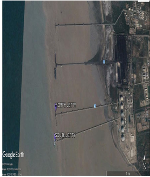
Fig. 2 Location of South and North Jetties of M/s PLL
