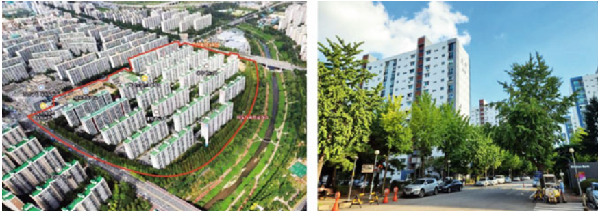
Fig. 2 Hanbo Mido Mansion apartment complex (1983). Source Naver Map Aerial Photography ( www.map.naver.com ) (left image) and View of the HMM (©Soe Won Hwang) (right image)
