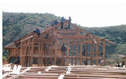
Building a new house in Muong Trai Commune. Photo by Dang, 2007
