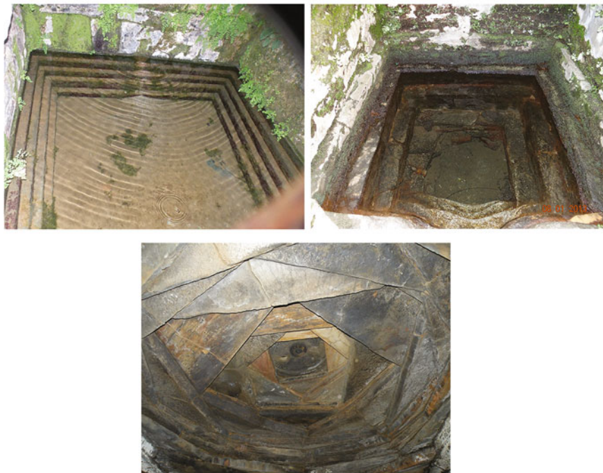
Fig. 7.3 Interiors of a Naula , steps leading to the tank (two pictures on the top) and the roof of the Naula (bottom picture)
