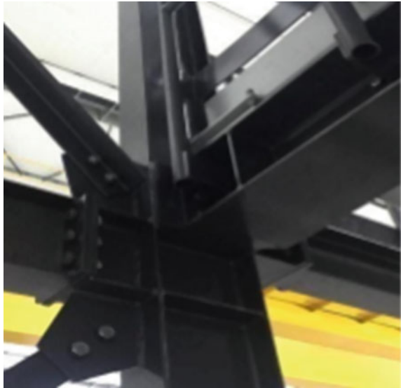
Fig. 12 Multiple connection joint
