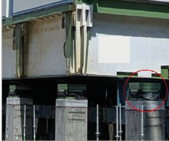
Fig. 9 Site photograph for bearing assembly module anchorage
