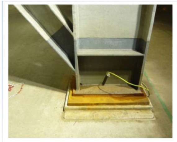
Fig. 1 Site photograph showing welding anchoring method
