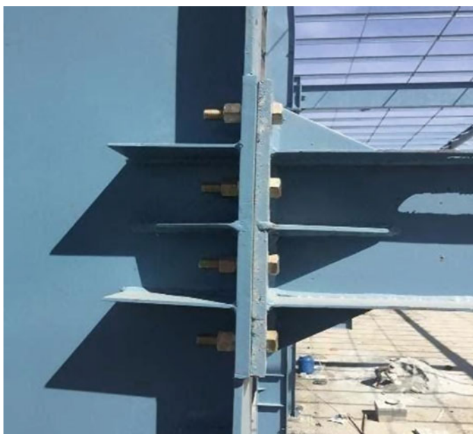
Fig. 10 Main beam to column connection
