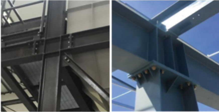
Fig. 13 Beam column connection
