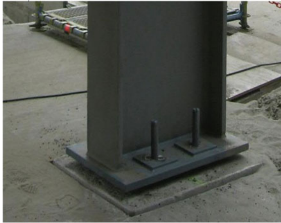
Fig. 6 Site photograph of coupler anchor bolts
