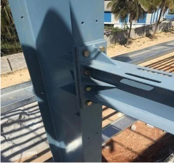
Fig. 11 Column to beam connection
