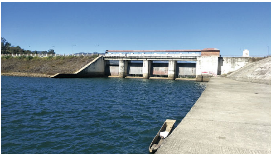
Fig. 1 Khuga dam and spillway
