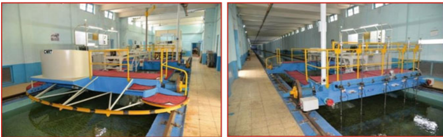
Fig. 1 Current meter rating facility at CWPRS
