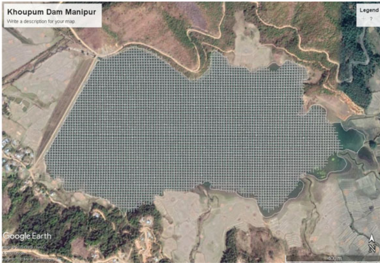
Fig. 1 Google image of Khoupum Dam boundary with data points
