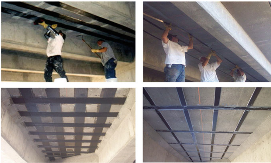
Fig. 3 External bonding of composites for strengthening of decks
