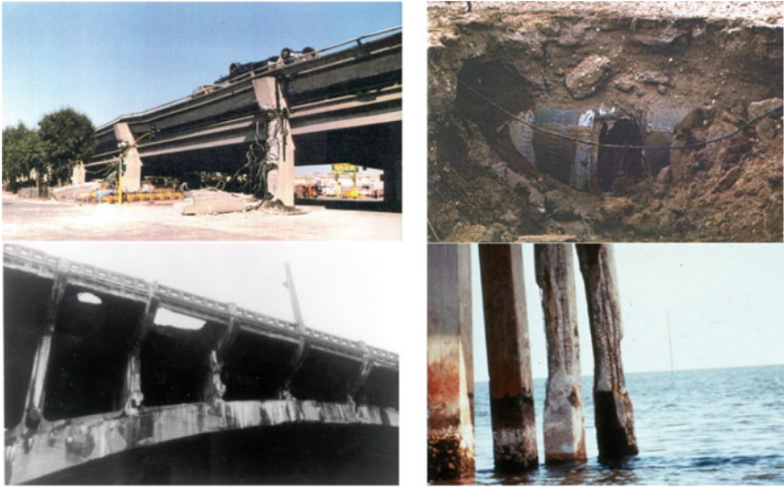
Fig. 1 Deterioration in infrastructure components
