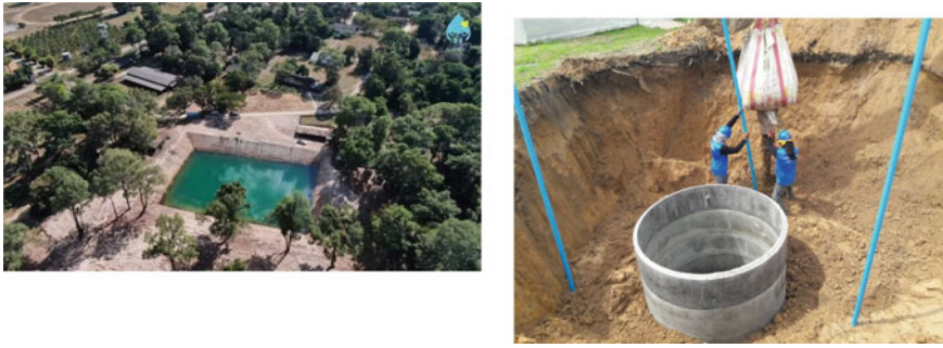
Fig. 3.3 Artificial groundwater recharge pond
