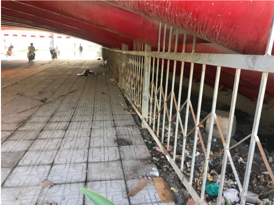
Fig. 8 Open space under Cong Ly Bridge, HCMC (Authors, 2019)
