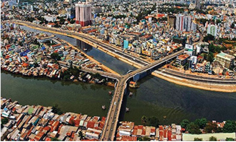
Fig. 1 District 8 and its iconic Y bridge (Source I Tour Vietnam [ https://www.itourvn.com ])
