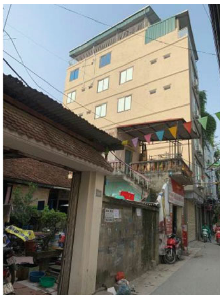
(f) Newly-built house
