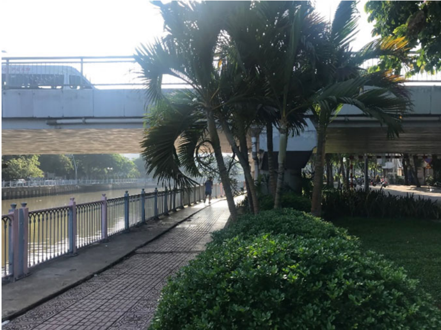
Fig. 10 Space along the canal under Hoang Hoa Tham Bridge, Phu Nhuan district, HCMC (Authors, 2019)
