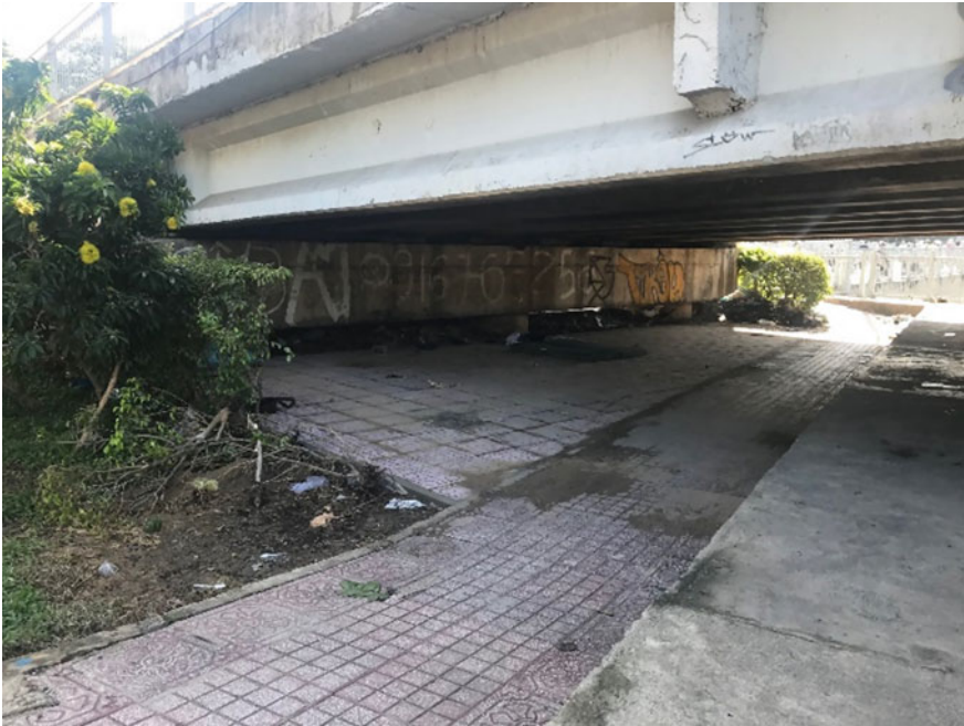
Fig. 6 Space under Bui Huu Nghia Bridge, HCMC (Authors, 2019)
