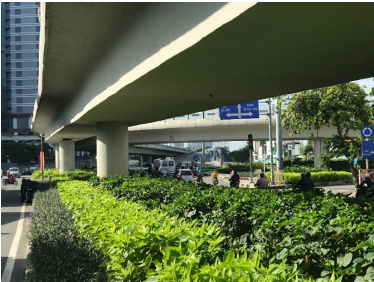
Fig. 12 Appealing design under Thu Thiem Bridge, HCMC (Authors, 2019)
