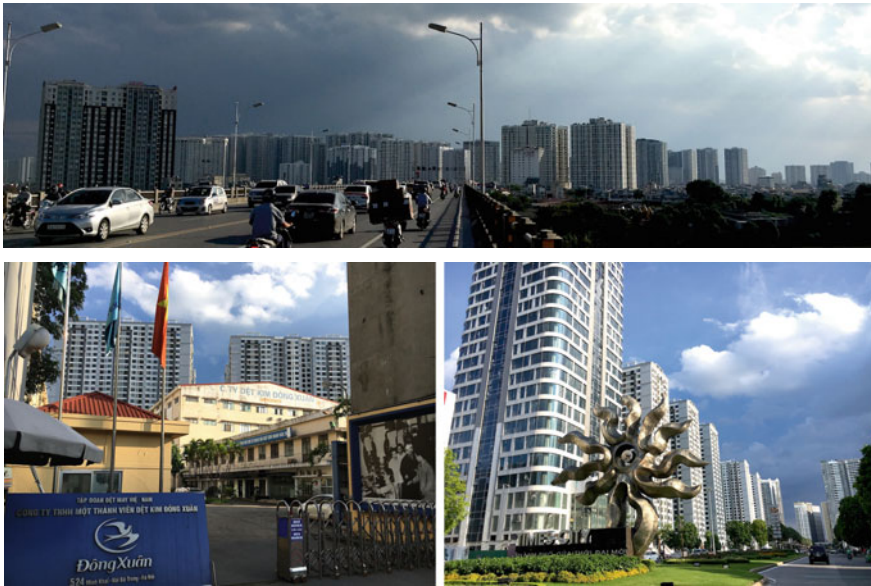
Fig. 5 Vinhomes Times City project: the changing skyline of Hanoi due to urban renewal (Source Authors)
