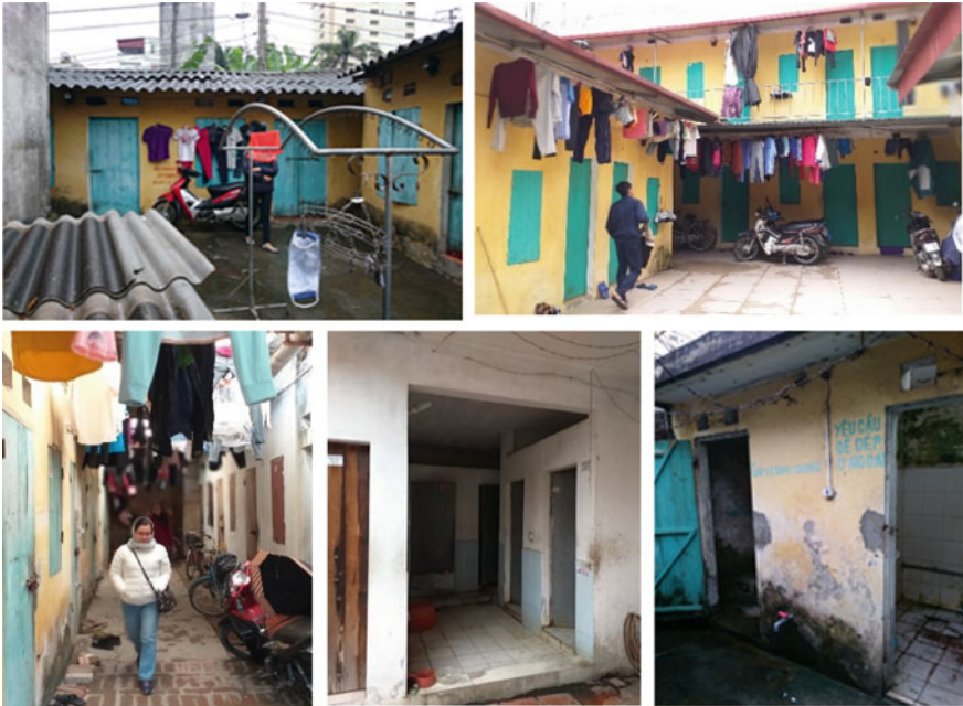
Fig. 3 Some pictures of village-based rental housing for workers near North Thang Long industrial zone. Source Authors
