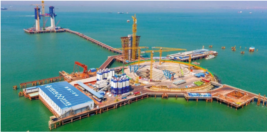
Fig. 2 Photo of structure layout in east anchorage area
