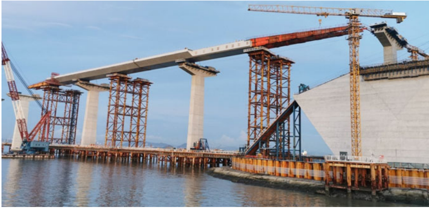
Fig. 8 Large section jacking of steel box girder
