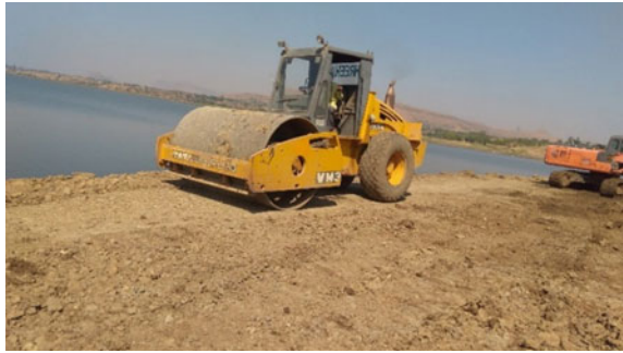
Fig. 7 Roller compaction of soil filled on upstream side
