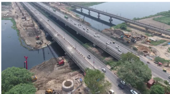
Photo 1 Bird's eye view of bridge during construction
