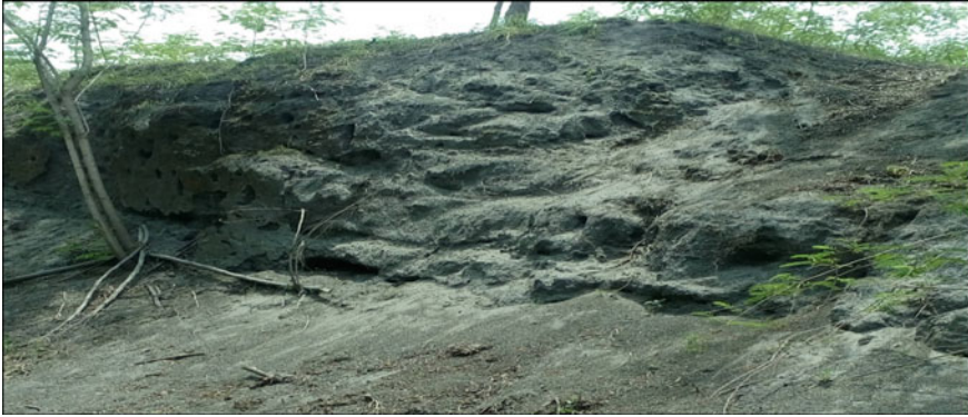
Fig. 2 Fly ash inside plant boundary
