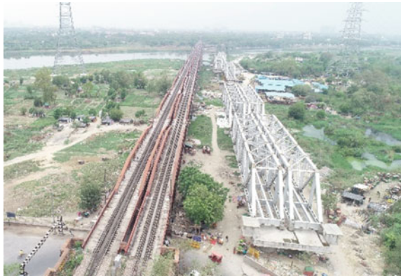
Photo 5 Drone view of new under construction bridge & old Bridge
