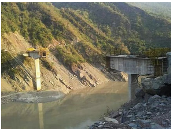
Photo 6 Portion of structure completed in 2010, before the work was suspended
