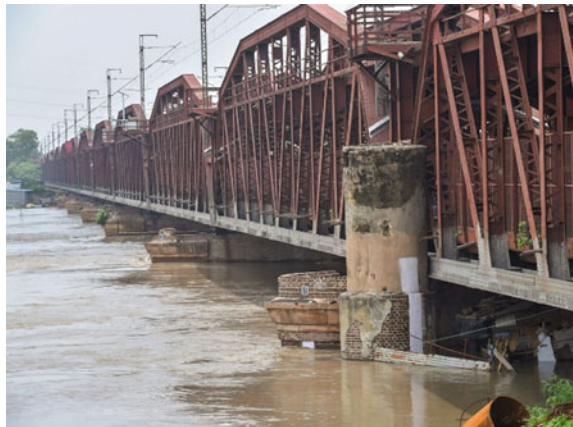
Photo 3 Existing 150 year old rail cum road bridge
