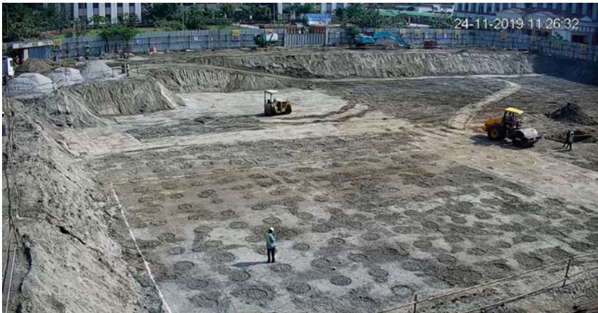
Fig. 5 Stone columns after installation at Tezpur site
