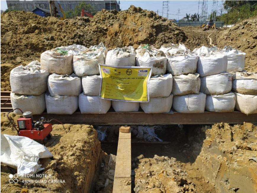
Fig. 9 Typical routine stone column load test arrangement
