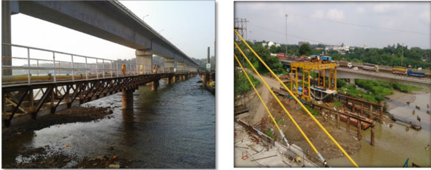
Fig. 5 Typical photograph showing temporary walkway and load out jetty
