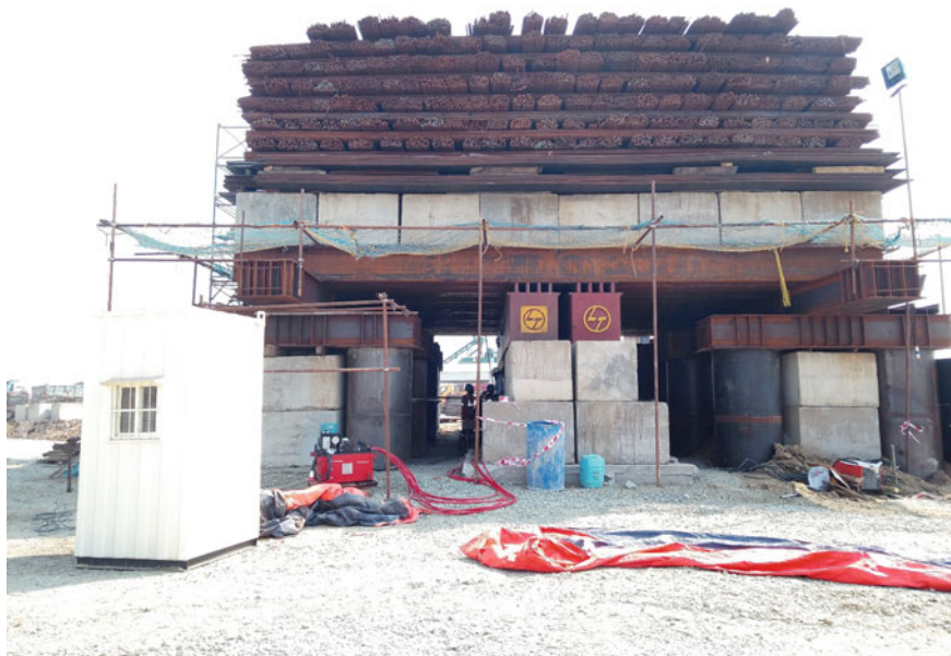
Fig. 6 Load test arrangement using liner pile as support to kentledge
