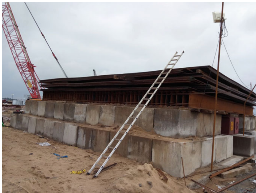
Fig. 3 Load test arrangement in site using concrete blocks
