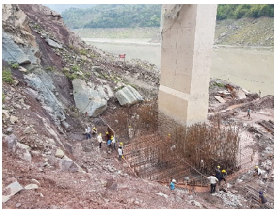
Photo 9 Casting of pile cap in progress at P2
