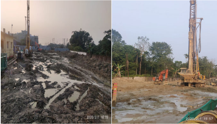
Fig. 4 Typical crane setup by dry bottom feed method (Courtesy: Keller)
