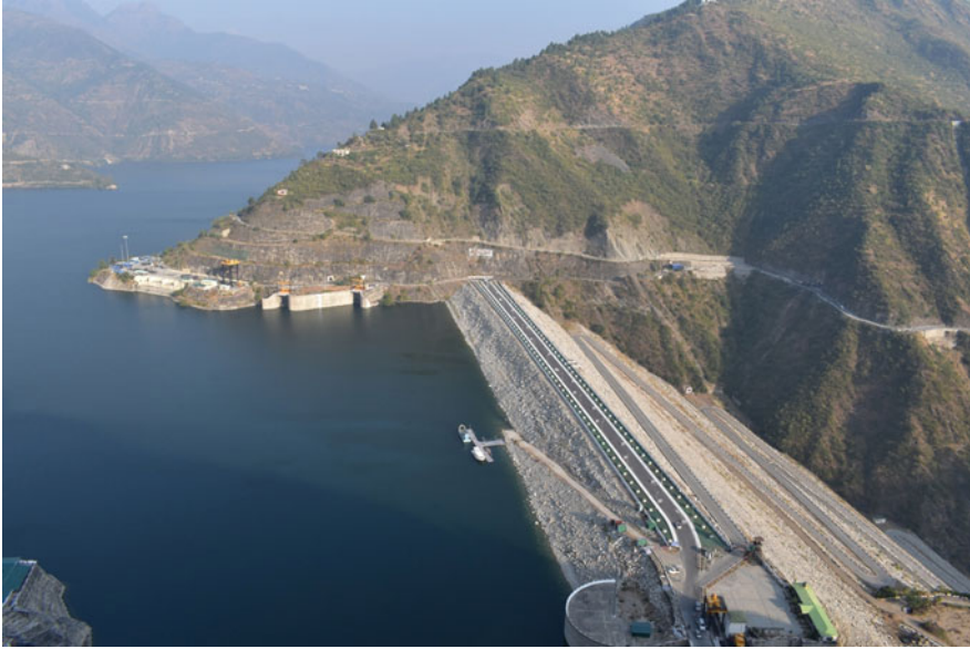
Fig. 25.3 The Tehri dam in Uttarakhand, India
