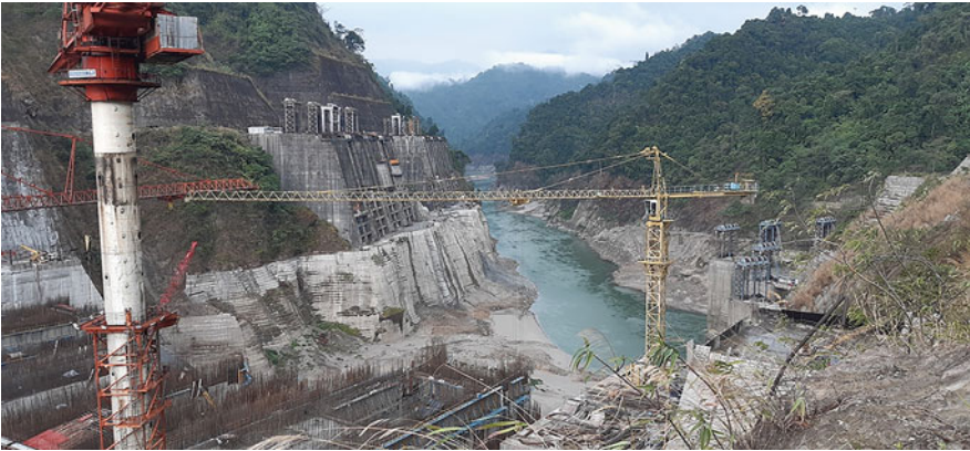
Fig. 25.4 The upcoming 2000 MW hydropower project in Subansiri, Arunachal Pradesh, India
