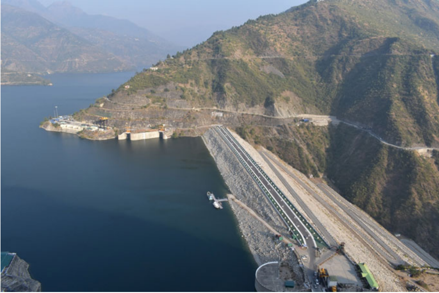
Fig. 25.3 The Tehri dam in Uttarakhand, India
