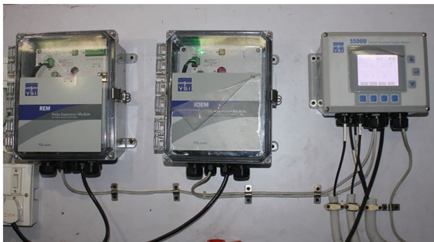
Fig. 11.10 Real-time DO monitor and alarming system (YSI 5500D) used at ICAR-DCFR, RAS facility at Bhimtal
