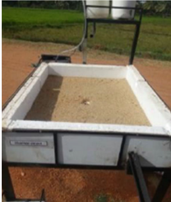
Plate 6.3 Laying of a sand layer under the solar still
