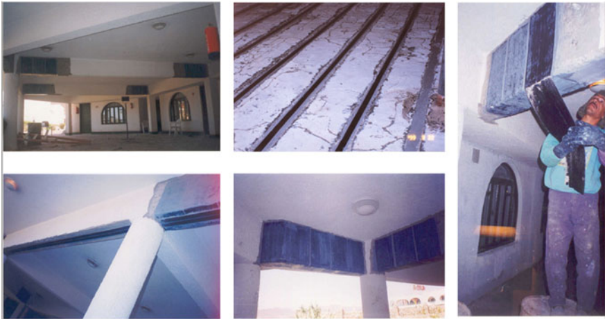
Fig. 5.16 Strengthening of the superstructure with CFRP
