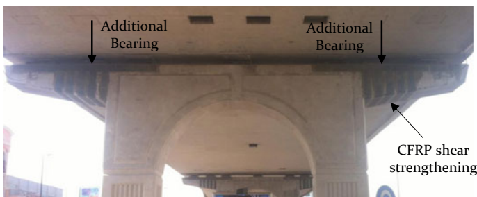
Fig. 3.26 Bridge pier after strengthening
