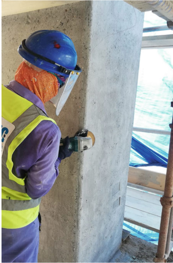
Fig. 2.9 Rounding column corners
