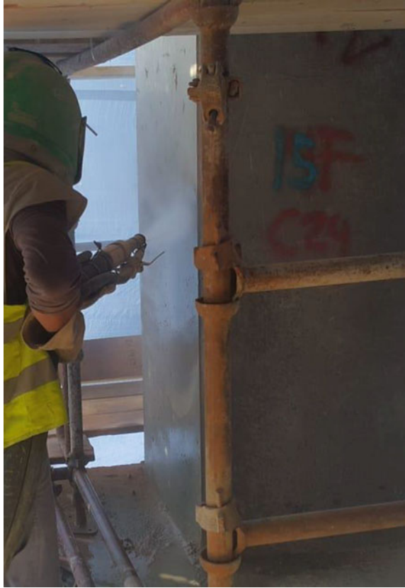
Fig. 2.8 Surface preparation of column
