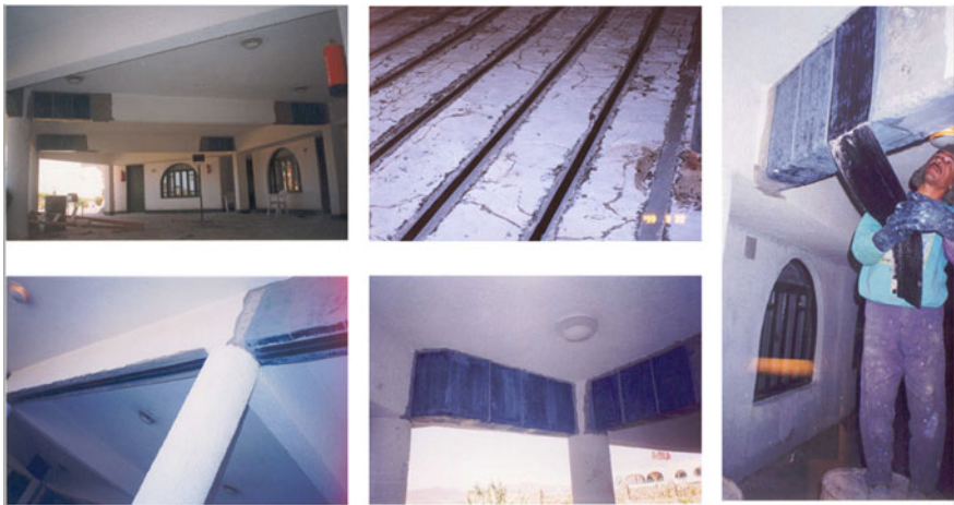
Fig. 5.16 Strengthening of the superstructure with CFRP
