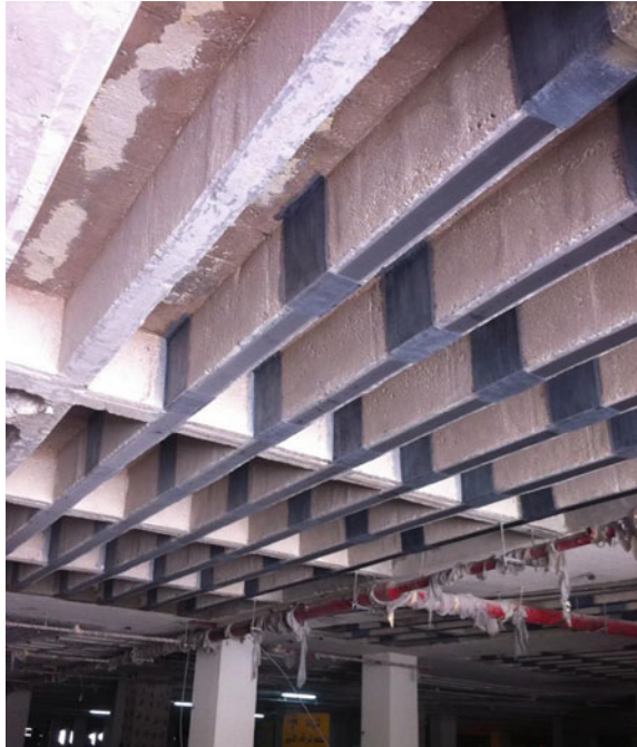
Fig. 3.8 Beam strengthening with externally bonded FRP
