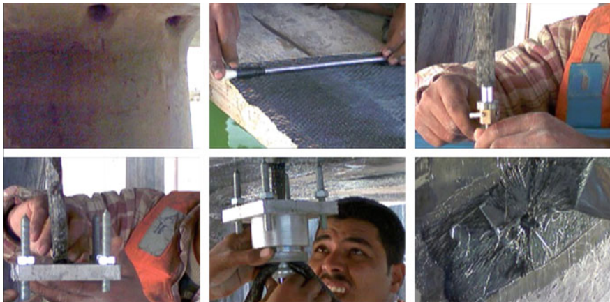
Fig. 6.9 Application steps of CFRP anchor
