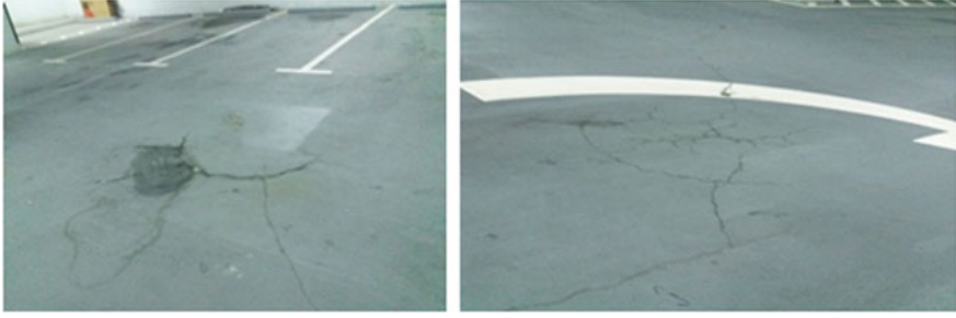
Fig. 5.8 Punching shear cracks in the raft
