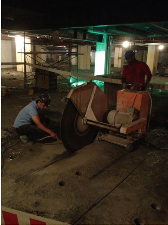
Fig. 4.27 Cutting the slab
