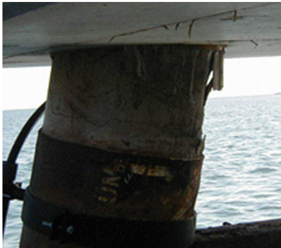
Fig. 6.5 Concrete crushing
