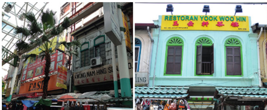
Fig. 4 Building façade hidden by trees and roofing structure/repainted shophouse
