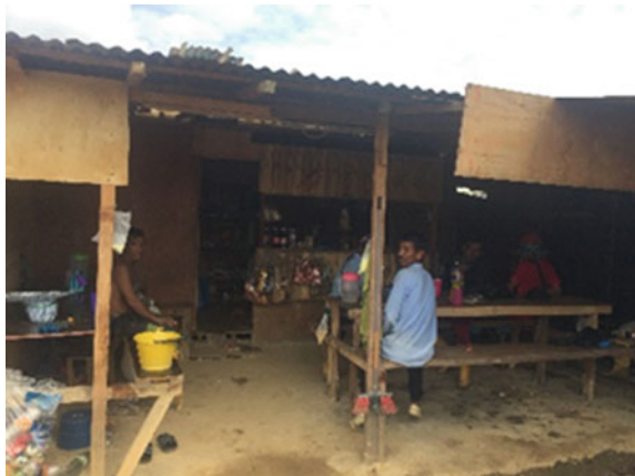
Fig. 5 Construction site B makeshift labourers canteen
