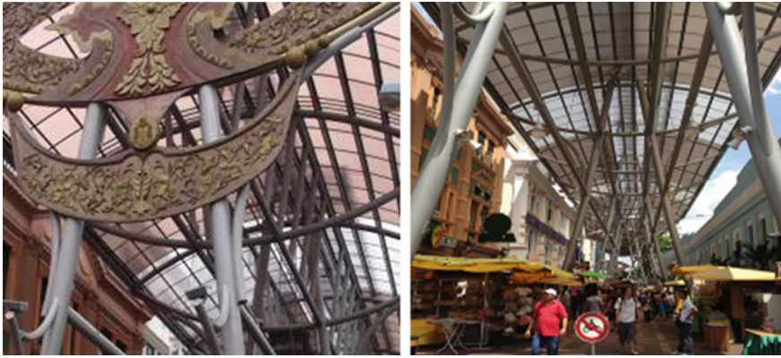
Fig. 9 Details on the roofing structure. Environment under roofing structure
