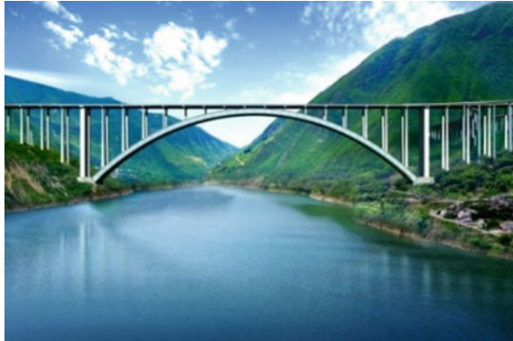
Fig. 6 Xining River Bridge
