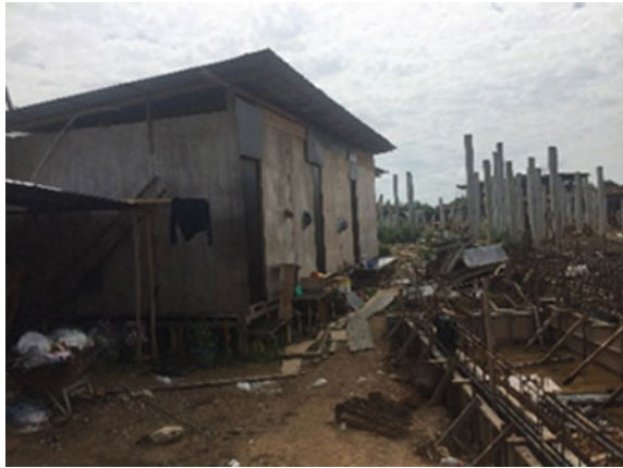
Fig. 4 Construction site B workers' quarters sited on one corner of the construction site
