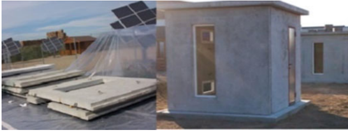
Fig. 6 Cubicles made of prefabricated concrete panels [53]
