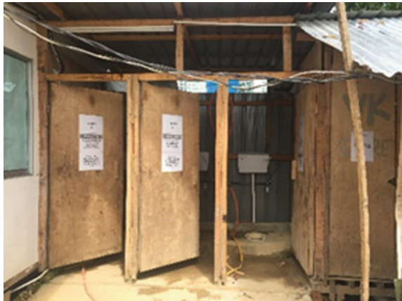
Fig. 7 Construction site C workers' quarters' utility cables hanging lowly across the quarters
