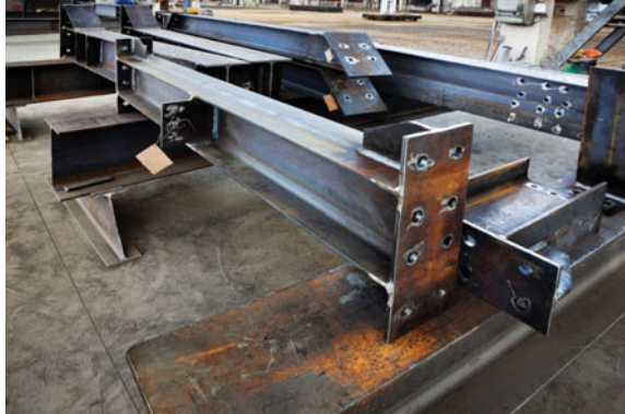
Fig. 8.2 The column fabricated at the yard (before painting)
