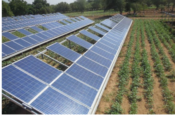
Fig. 22.5 Agrivoltaic system installed at ICAR-Central Arid Zone Research Institute, Jodhpur
