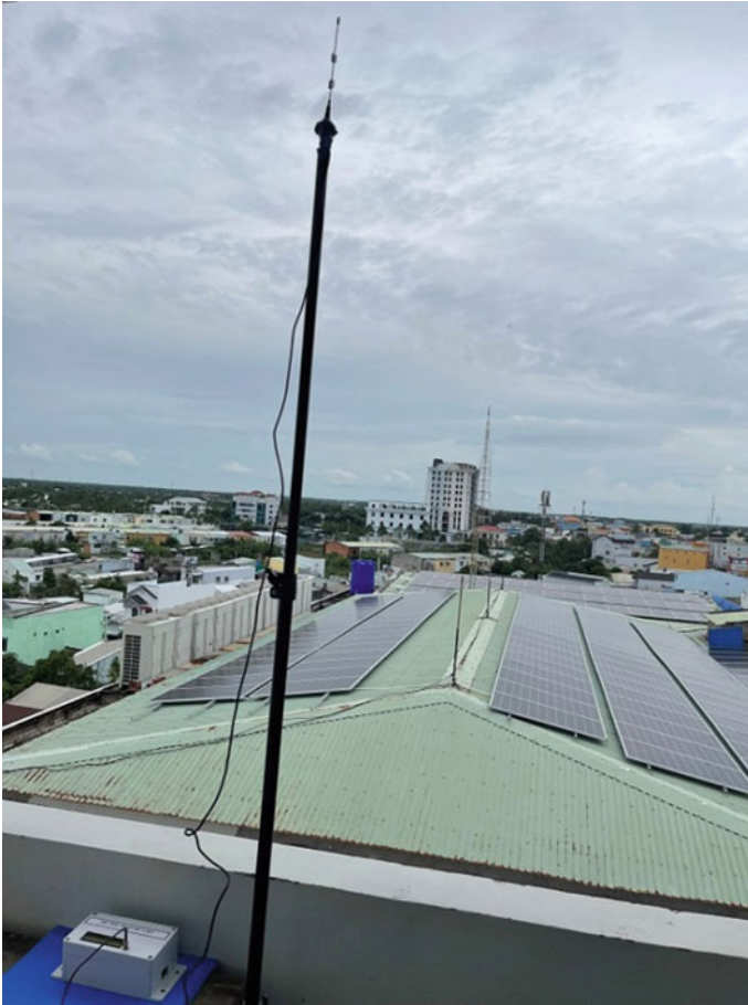
Fig. 12 Installation of Gateway station
