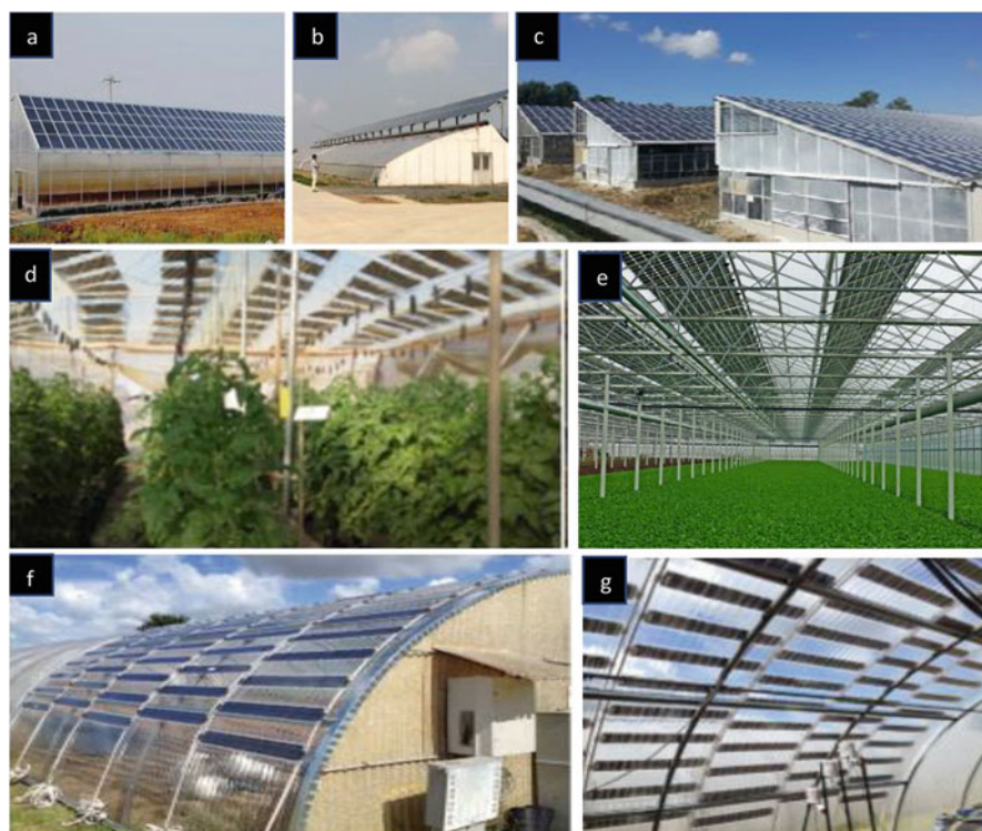
Fig. 4 Possible field arrangements of PV panels (a–c) opaque PV modules (Xue, 2017; Cossu et al., 2016a), (d, e) continuous rows (Ezzaeri et al., 2020; Allardyce et al., 2017), (f, g) checker-board (Marucci et al., 2018)
