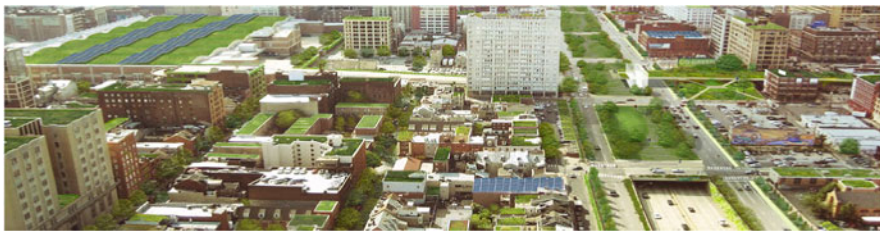
Fig. 4.2 Green storm water infrastructure in Philadelphia (USA). ( Image Courtesy: Philadelphia Water Department )
