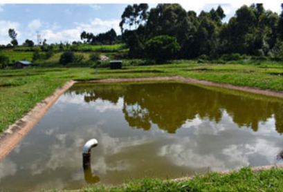
Concrete ponds Source: Author
