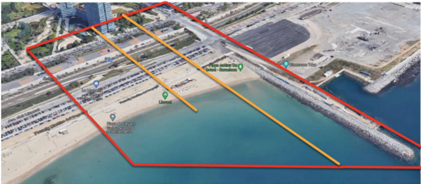
Fig. 2.3 Work area for the visit (Forum). (Source Google Maps, edited by the authors)
