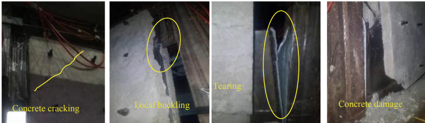
(c) Deformation and damage of the BRSW-3
