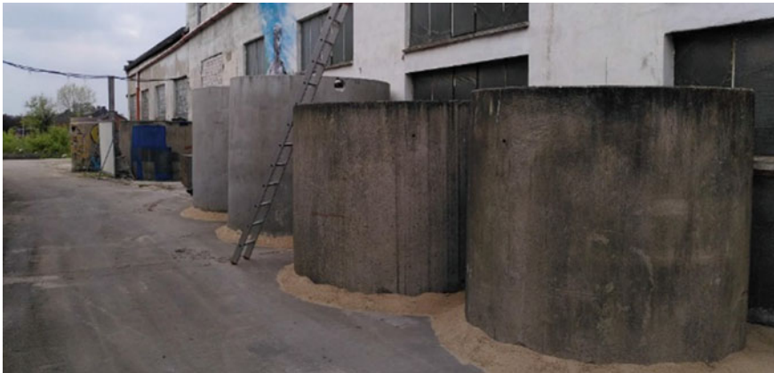
Fig. 5 Small sewage treatment plant
