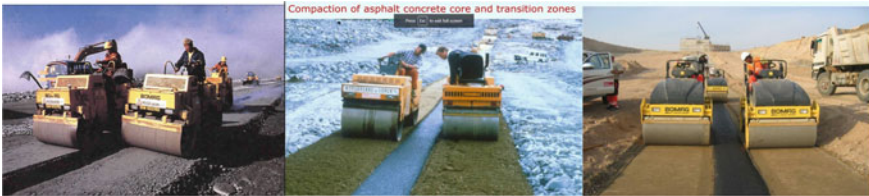
Fig. 29.5 Simultaneous compaction of core and filter [4]
