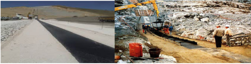
Fig. 29.1 Asphaltic core in dam (Styggevatn Dam, Norway, [4])
