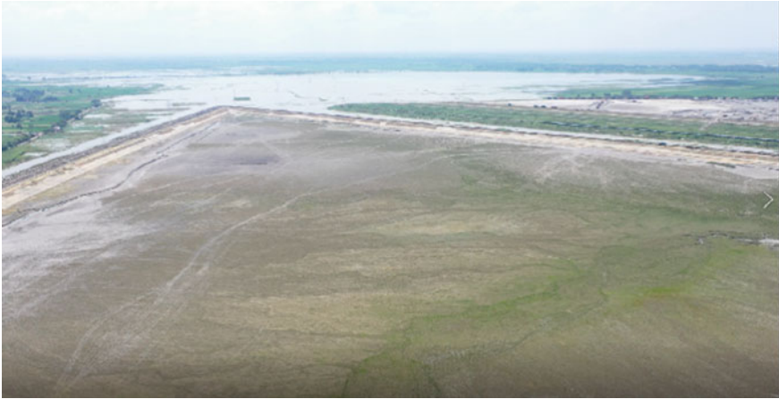
Fig. 41.1 Inside area of ash pond in 1st raising
