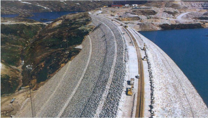
Fig. 29.9 Storglomvatn Dam (125 m), Norway [8]
