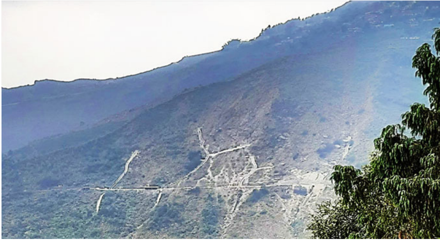
Fig. 16.1 Failed slope face (2021)
