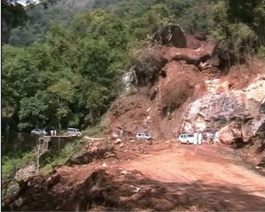
Fig. 12.1 Road damage due to Marappalam slope failure (Senthilkumar et al. [5])
