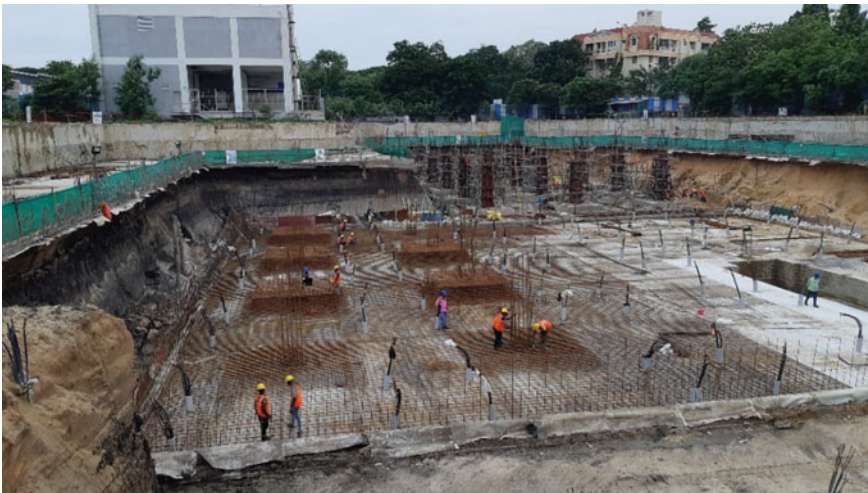
Fig. 28.5 Site view showing passive berm and raft construction
