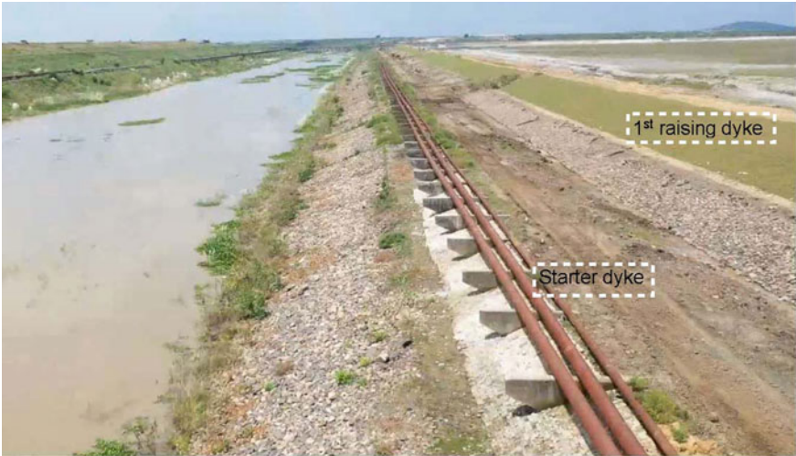
Fig. 41.2 Downstream side view of ash pond
