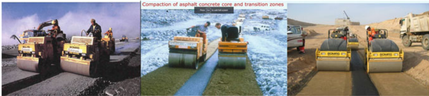
Fig. 29.5 Simultaneous compaction of core and filter [4]
