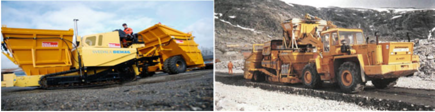
Fig. 29.4 Asphalt core placing machine (paver) [4]
