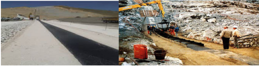
Fig. 29.1 Asphaltic core in dam (Styggevatn Dam, Norway, [4])
