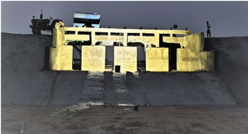
Fig. 41.6 Upstream view of re-constructed spillway in dyke embankment
