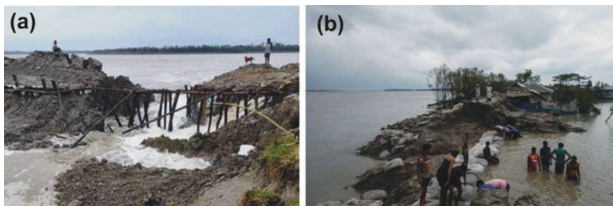
Fig. 7.2 (a–b) Devastative floods at Indian Sundarbans caused by massive failure of manmade embankments during severe cyclonic storm disasters during (a) Super Cyclone “Amphun,” May—2020; (b) Cyclone “Yash,” May—2021
