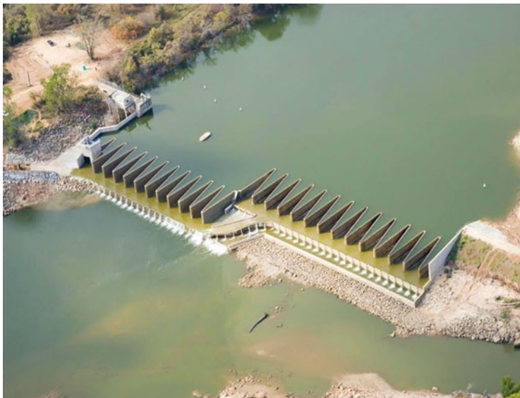
Fig. 8.3 Triangular Labyrinth Weir (Tunc and Emirođlu 2018)
