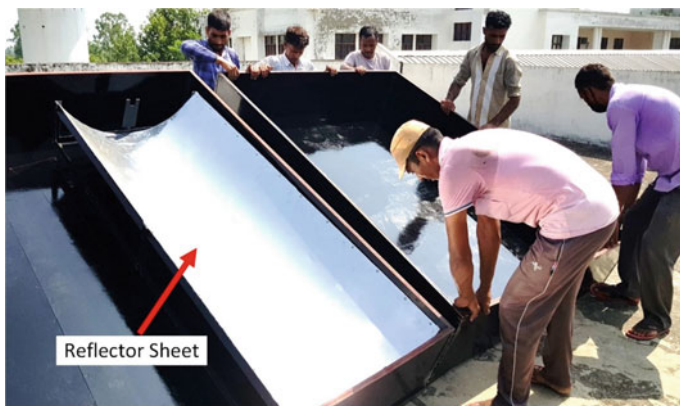
Fig. 2 Installation of the experimental setup
