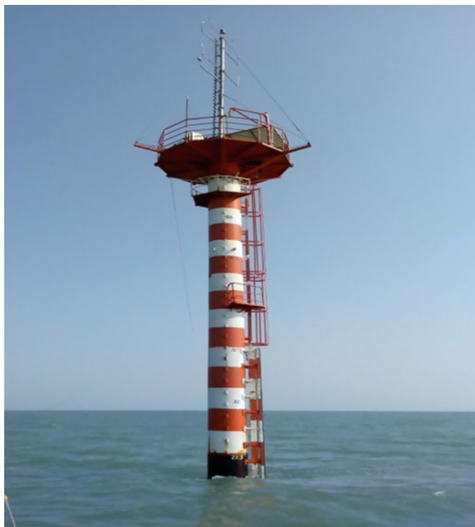
Fig. 9 LIDAR-based based platform in Gulf of Kutch installed by MNRE and NIOT (Vedachalam et al. 2018; Raju et al. 2020)
