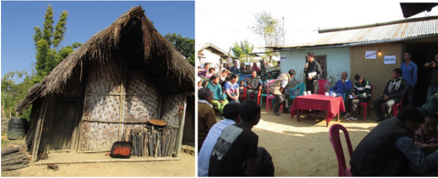
Fig. 2 A tilted hut at Kabuikhullen village in the epicentral region of the 2016 Tamenglong earthquake. Right panel shows a meeting and counselling of the villagers
