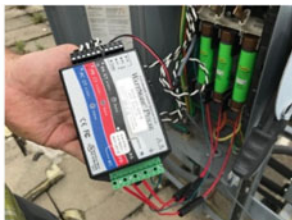
(b) Power Sensors for ODU
