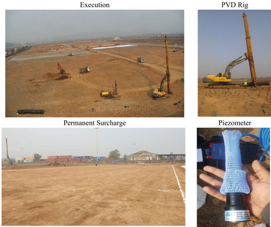
Fig. 7.3 Execution images of PVD and surcharge
