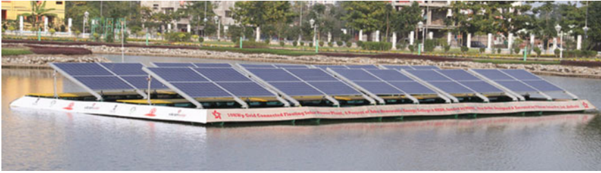
Fig. 5 Floating solar PV of 10 KWp capacity in Kolkata [16]
