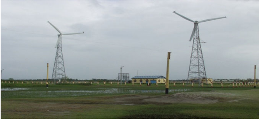
Fig. 7 2 MWp wind farm at Frasergunj in West Bengal [19]
