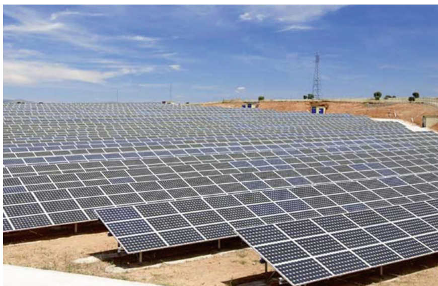
Fig. 4 5.5 MWp power plant at Salboni in West Bengal [15]
