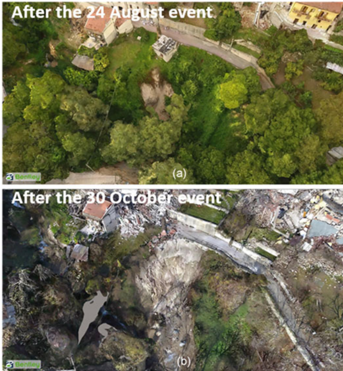
Fig. 32 3D model of the failure observed in area #5 in Fig. 28 following: a the 24 August and b the 30 October event (modified from GEER 2017)
