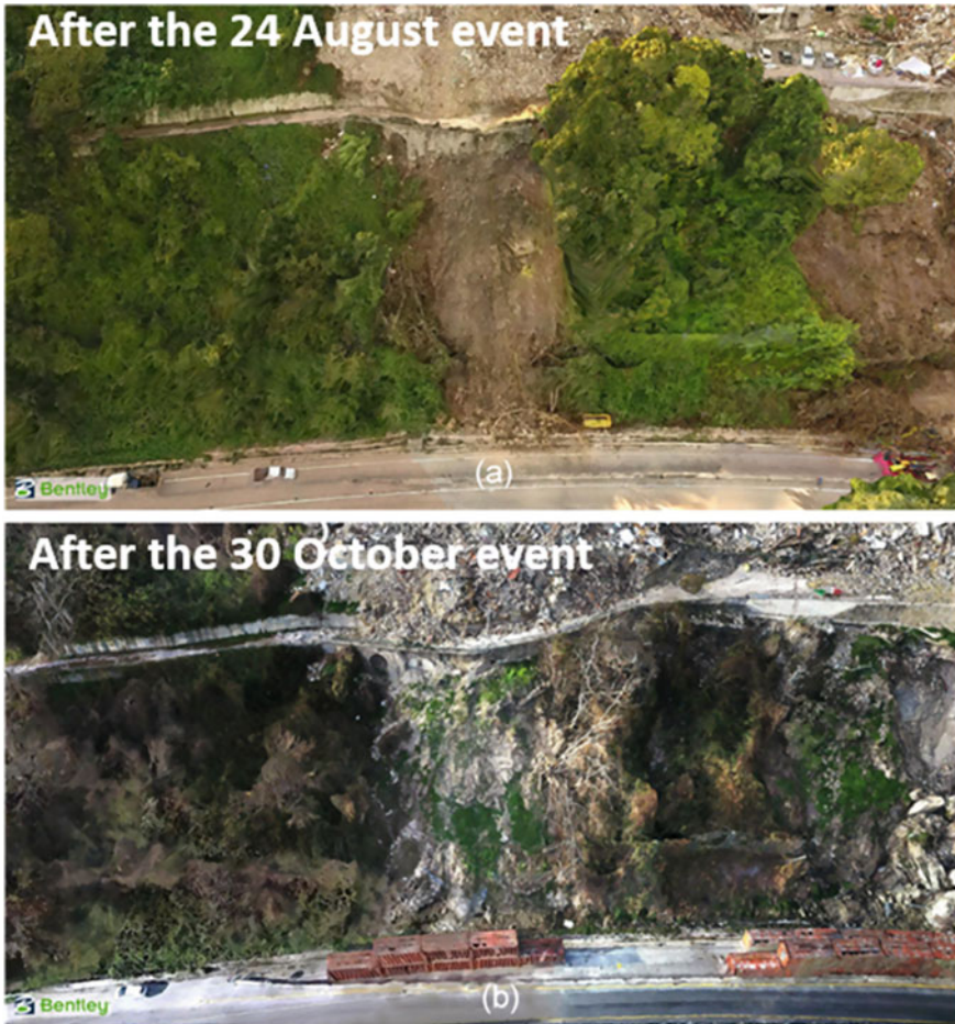
Fig. 30 3D model of the landslide #2 in Pescara del Tronto following: a the 24 August and b the 30 October event (modified from GEER 2017)
