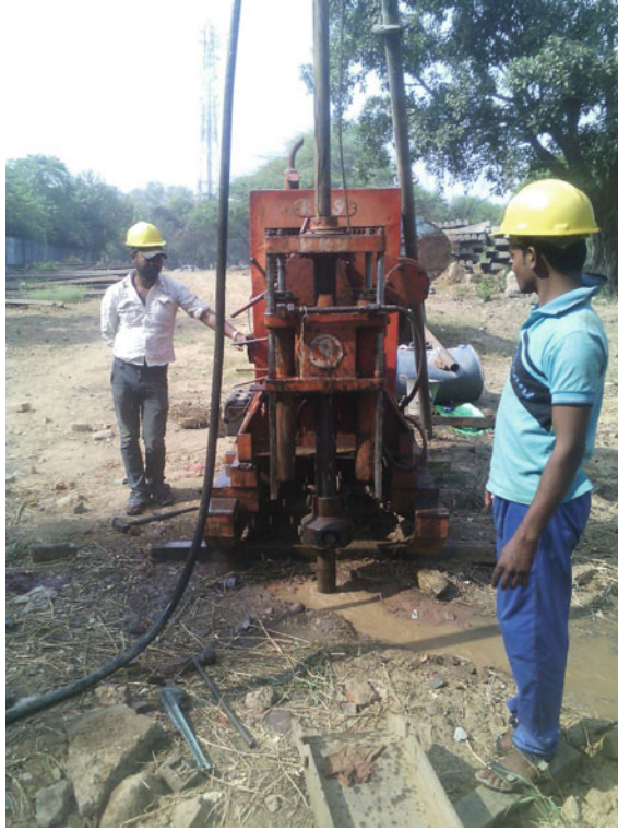
Fig. 18.2 Borehole drilling in progress
