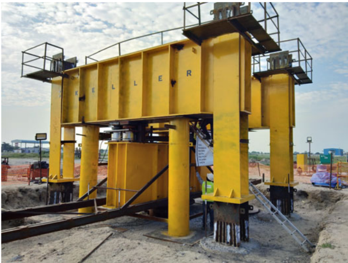
Fig. 23.3 Actual load test setup at site
