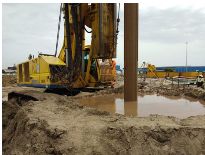
Fig. 23.6 Drilling of boreholes using hydraulic rig
