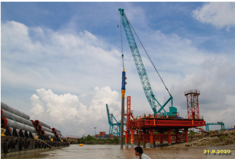
Fig. 29.3 Diesel or hydraulic hammer
