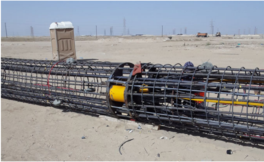
Fig. 2.2 BDSLT pile installation
