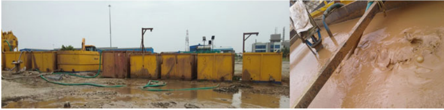
Fig. 23.4 Bentonite tank setup
