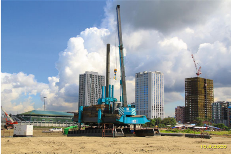
Fig. 29.2 Silent pile driver
