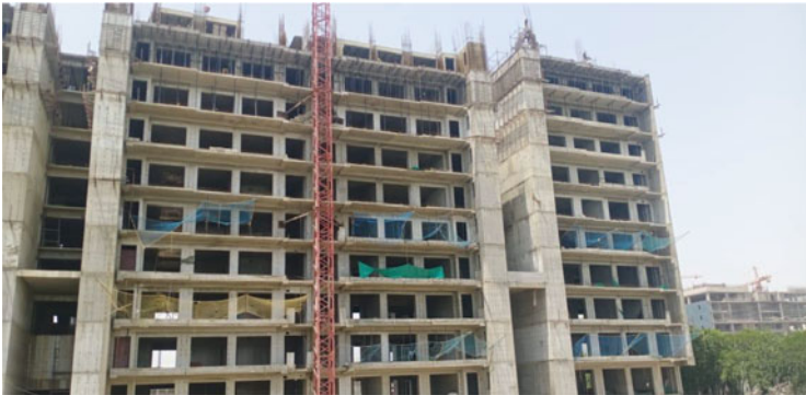
Fig. 9.13 Building under construction
