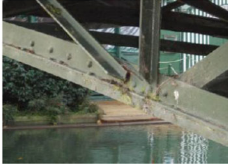
Fig. 14 A, hogging of the underneath bridge structure. B, Shear cracks due to abutment rotation observed at the Antigua Street Footbridge Source (Palermo et al. 2011)
