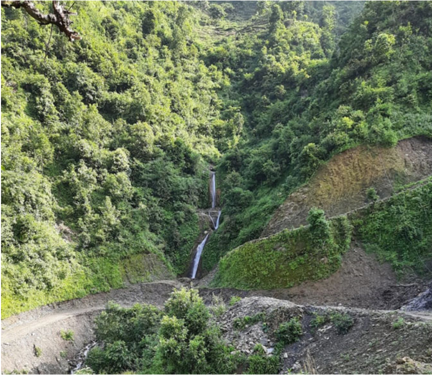
Fig. 3 Soil erosion from the newly constructed rural road in Kosrang. (Courtesy Ganesh Dhungana)
