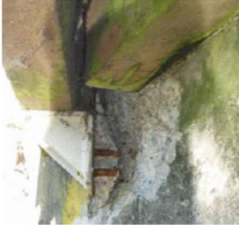
Fig. 14 A, hogging of the underneath bridge structure. B, Shear cracks due to abutment rotation observed at the Antigua Street Footbridge Source (Palermo et al. 2011)
