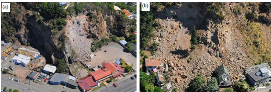
Fig. 6 Rock falls and sliding on the Port Hills Source (Cubrinovski et al. 2011)
