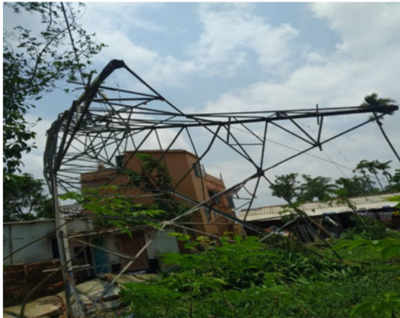
Fig. 8 Completely damaged Transmission Tower due to the shear failure of connection
