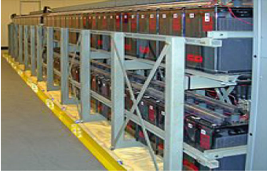
Fig. 3 A bank of batteries in a large data centre used to provide power until diesel generators can start [7]
