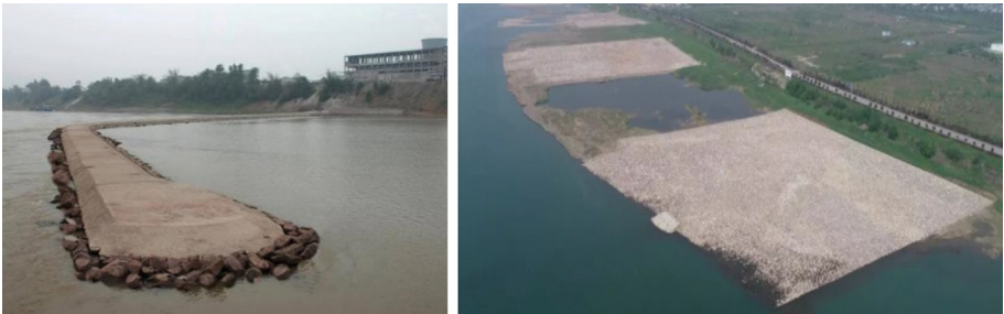
Fig. 3. Classic river training works (left: spur dike; right: flexible mattress belt).
