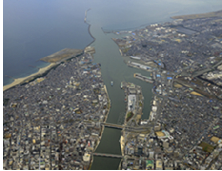
Fig. 2. Aerial photo of the port area.
