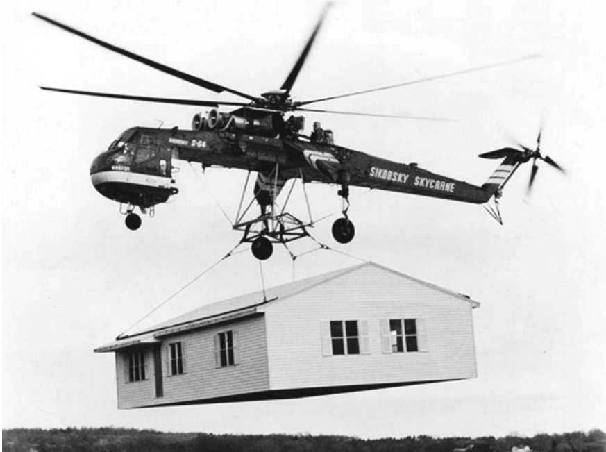
Fig. 3 A Sikorsky Skycrane carrying an accommodation
