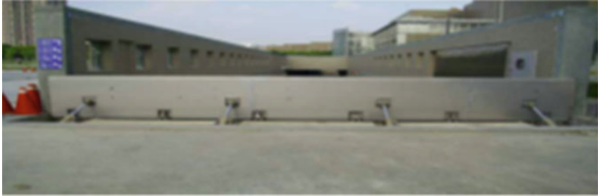
Fig. 3 Auto-flip flood wall barrier (Source Delta Technology [6])
