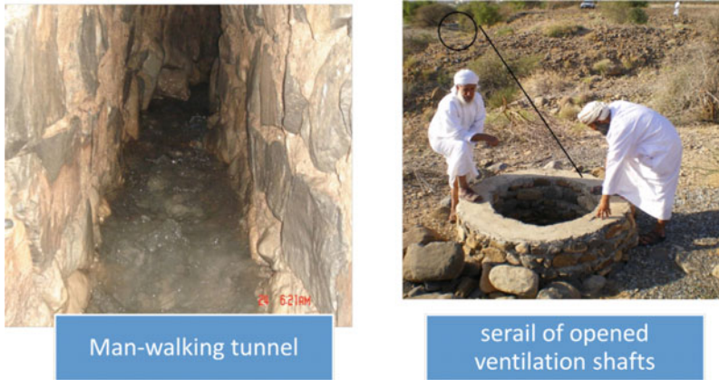
Fig. 2 Field survey constructed daudi identified components. The picture (left side) indicated a man-walking tunnel for falaj al-khatmeen in the district of burkat al-mouz (approximately 2,450 m long with a two-meter width and one meter height), as indicated above. The second picture (right site) shows author viewing, along with falaj al-malki wakeel (administrative agent), a one ventilation shaft which deeply is attached to the tunnel forming a horizontal tunnel attached with serial of these shafts. The main function of these is to allow air inside the tunnel and also as a means to get rid of the dirt from the tunnel construction, and later used as access for maintenance
