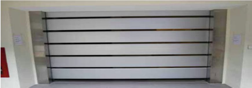
Fig. 6 Auto-stacking flood wall barrier (Source Delta Technology [6])
