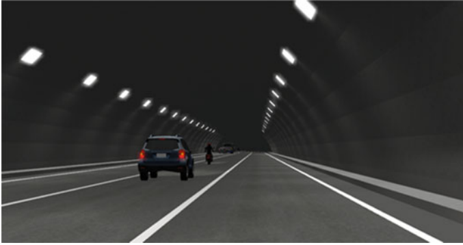
Fig. 5 One of the completed tunnel lighting system model
